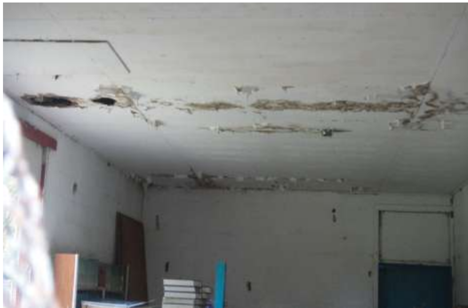
Source: Inspection team, December 14, 2010
