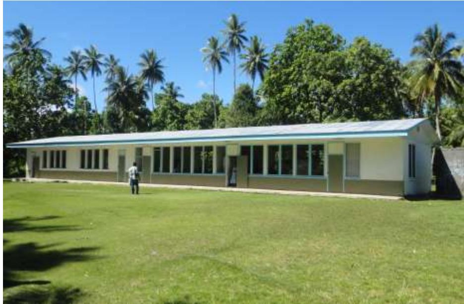
Source: Inspection team, December 14, 2010
